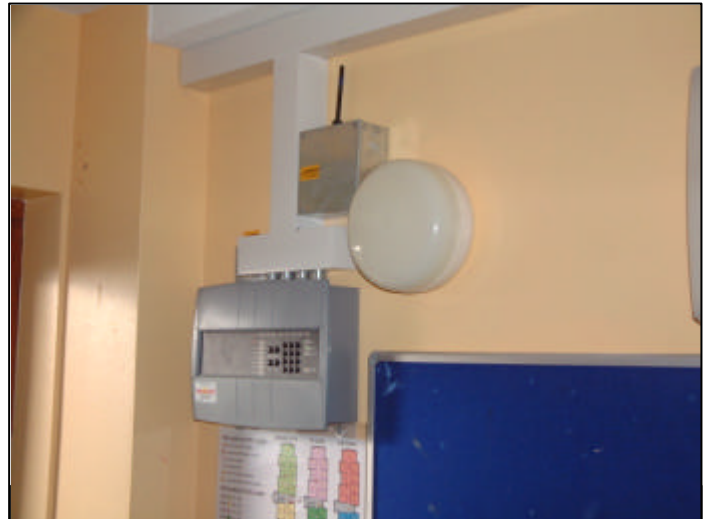
Each alarm is electronically linked to a radio that sends an alarm to the Safety Call Computer
